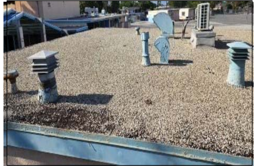
Deteriorated Roofing
