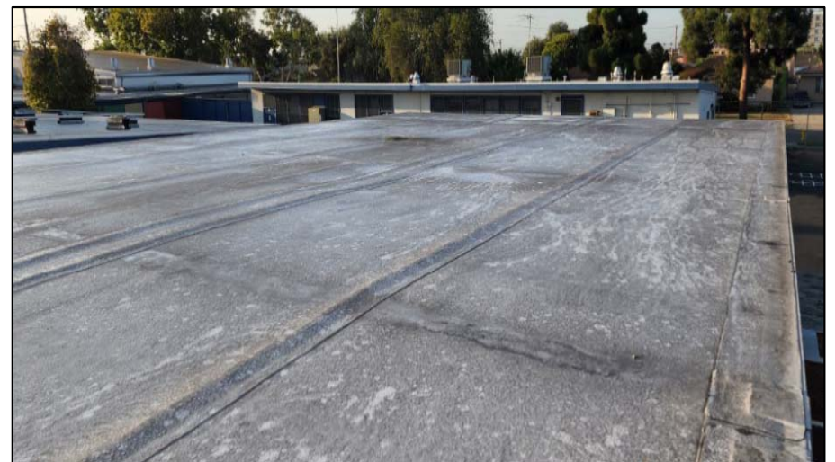
Deteriorated Roofing
