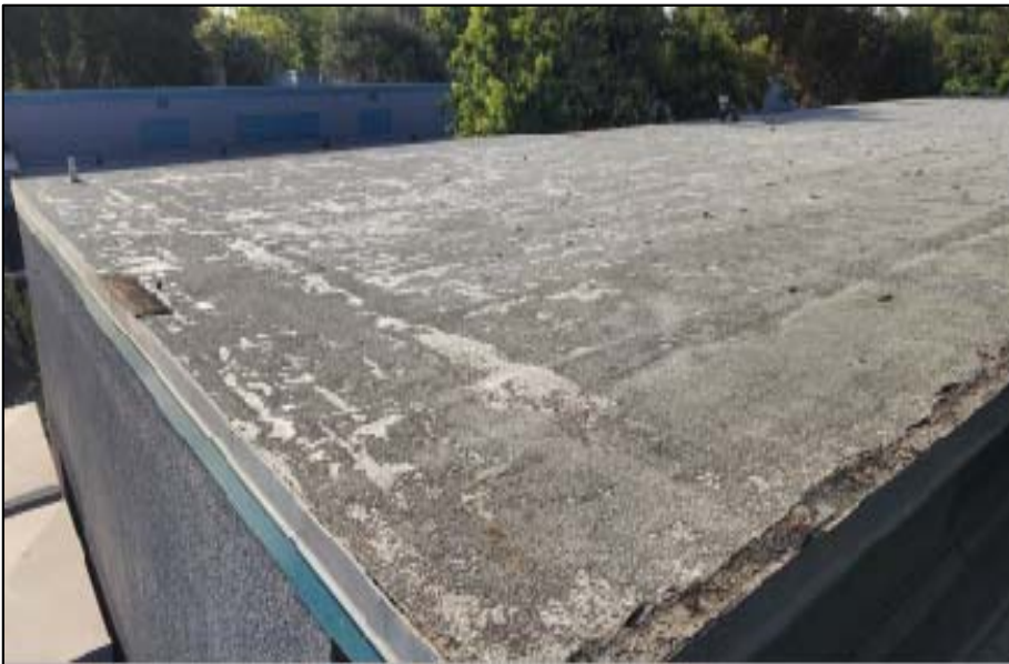
Deteriorated Roofing
