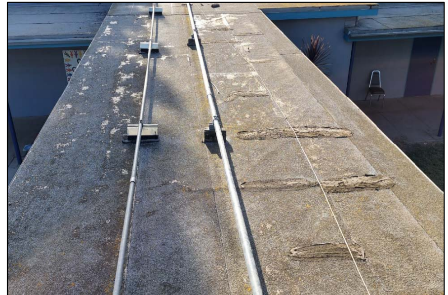
Deteriorated Roofing
