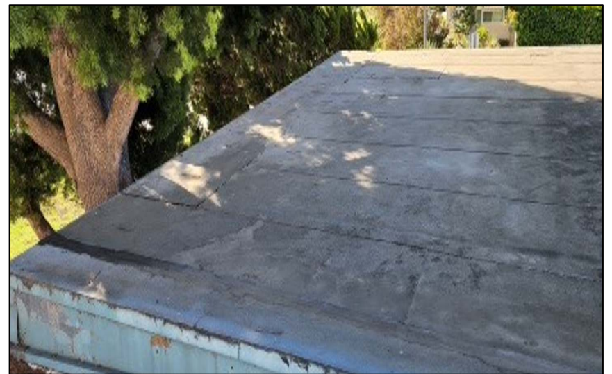
Deteriorated Roofing
