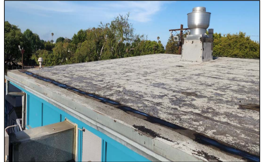
Deteriorated Roofing
