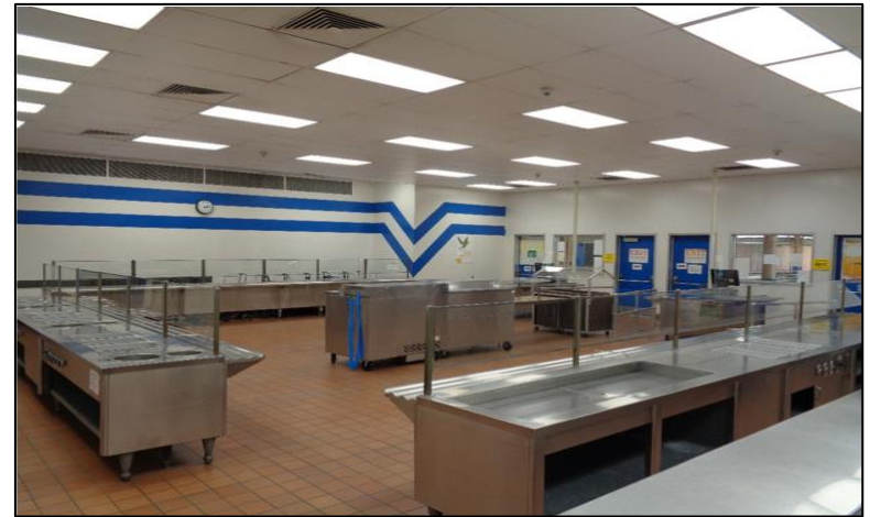
Obsolete Serving Line – Carnegie MS
