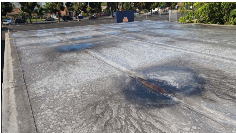
Deteriorated Roofing
