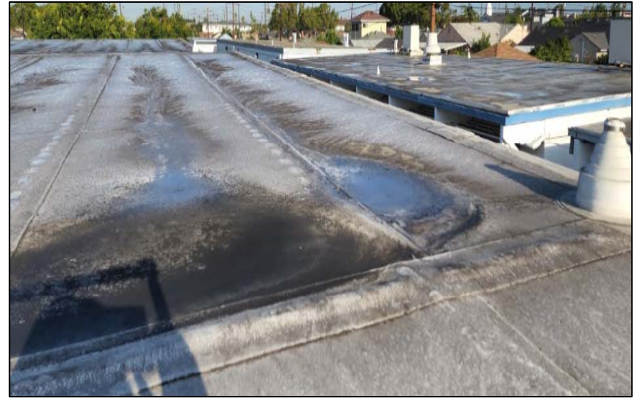
Deteriorated Roofing
